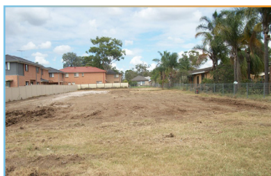
Above: The vacant site in Rooty Hill, 2010, prior to construction. Photo: SDN Archive
